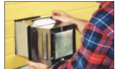
Install Vent Termination
